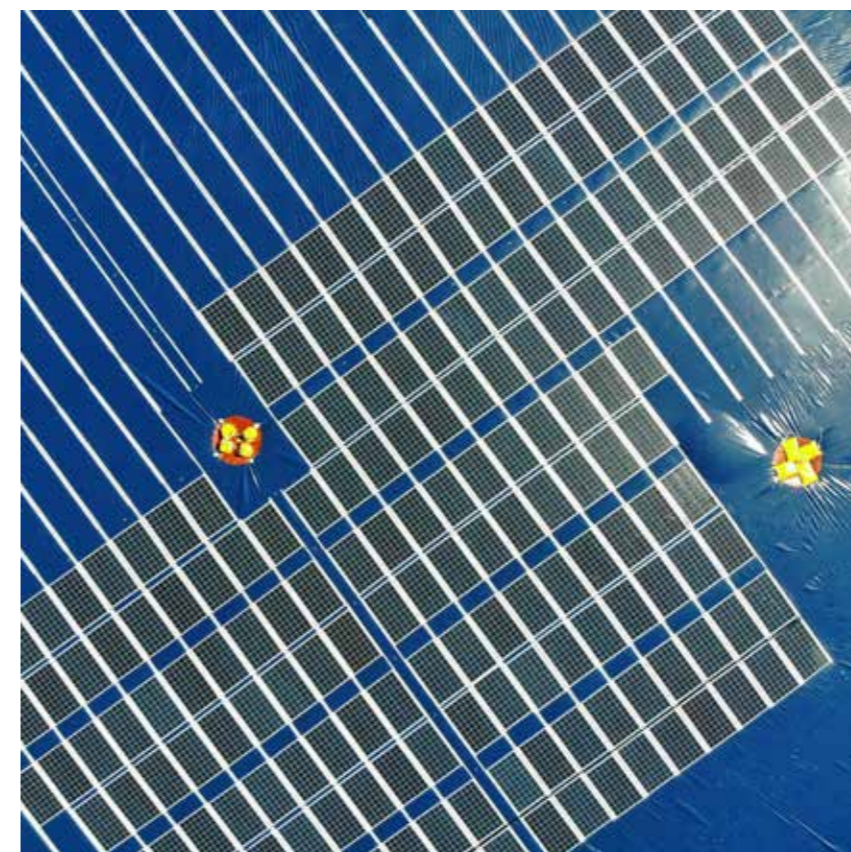
» Floating solar cell modules mounted on a polymer membrane: Photo: Ocean Sun
